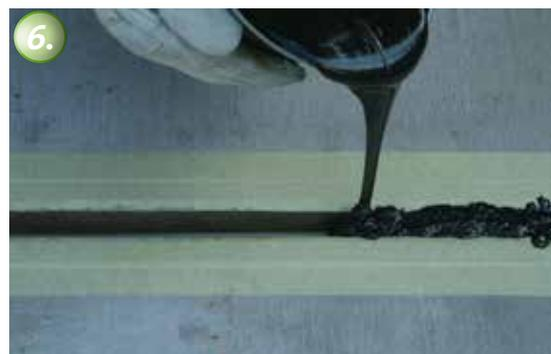
6. The joint is filled approximately 2 hours after applying the KÖSTER FS Primer 2C.
