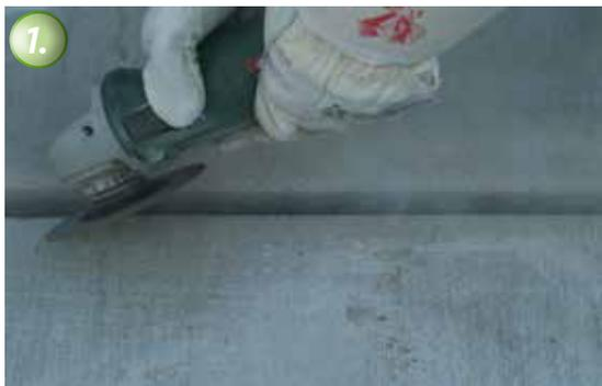
The joint flanks are beveled before the application of the Joint Sealant. The bevel must be at least 10 mm wide and in a 45° angle.
