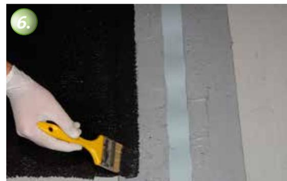
**6.** After KÖSTER KB-Pox Adhesive has cured for 24 hours, the area water-proofing can be applied overlapping onto the epoxy layer.
