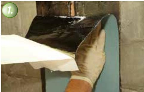
*The substrate is first primed, for example with KÖSTER KBE Liquid Film. After curing the KÖSTER Special Joint Tape is applied. KÖSTER Special Joint Tape is cold applied, self adhesive and is simple to use.*
