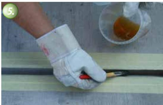
5. Absorbent substrates must be primed with KÖSTER FS Primer 2C twice. Non-absorbent substrates are primed once.
