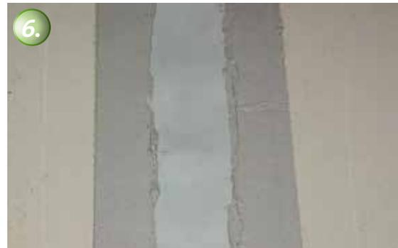
**6.** Remove the masking tape on both sides before the adhesive cures in order to achieve a clean finish.
