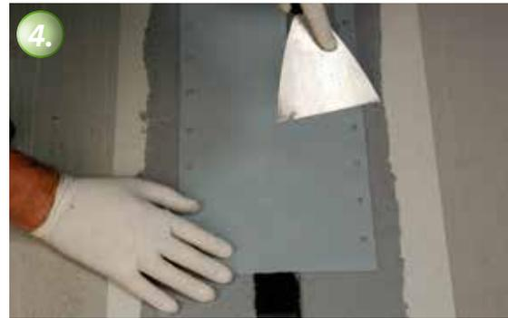
**4.** Press the KÖSTER Joint Tape onto fresh adhesive layer.
