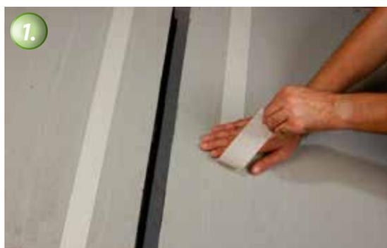
1. Initially both sides of the joint are masked with tape.
