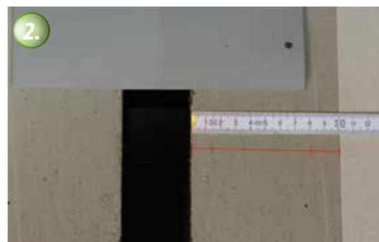
2. Embed KÖSTER Joint Tape 20 min. 4 cm (Joint Tape 30 min. 5 cm) into the adhesive on each side. The adhesive is applied 2 cm farther onto the substrate.
