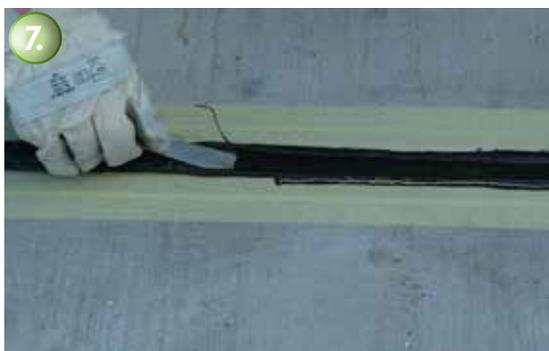
7. The Joint Sealant is smoothed, for example with a spackle. The tape should be removed before the Joint Sealant has hardened.
