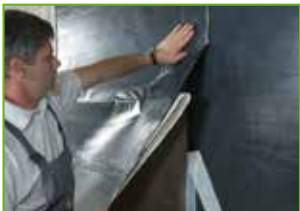
Applying the membrane
