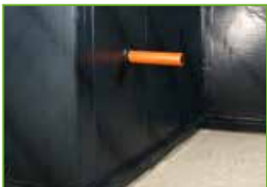
The waterproofing is installed.
