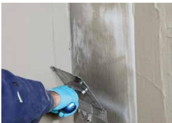
*Application of the first layer of KÖSTER NB Elastic grey to the wall with brush or trowel. KÖSTER Flex Fabric is embedded in the first layer.*
