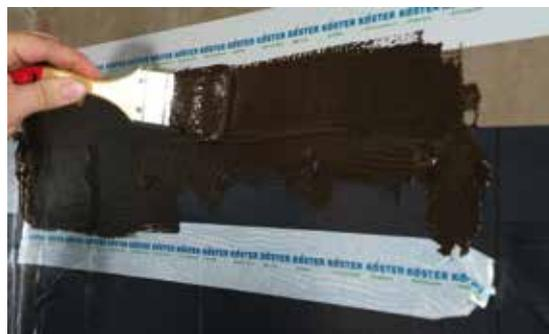
The edges of the membrane are sealed with KÖSTER KBE Liquid Film.
