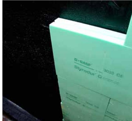
**Insulation boards can be easily attached with two-component KÖSTER PMBs. It is important the insulation boards are fully bonded.**
