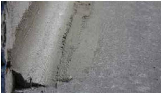
*Corners are rounded out with a fillet made from KÖSTER WP Mortar.*
