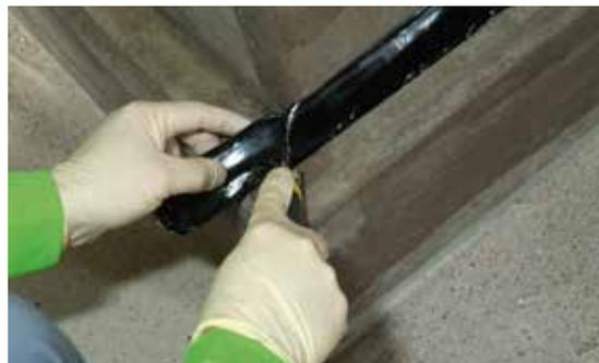
Fillets can be made of either KÖSTER WP Mortar or alternatively with the cold self-adhesive KÖSTER KSK Triangular Ribbon.
