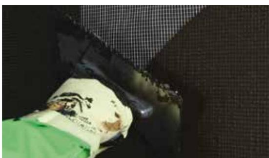
KÖSTER Glass Fibre Mesh is embedded into the first fresh layer of KÖSTER Deuxan® 2C. Generally, mesh is embedded in areas which are in danger of cracking. When waterproofing against pressurized water, KÖSTER Glass Fibre Mesh must be embedded in the entire area.
