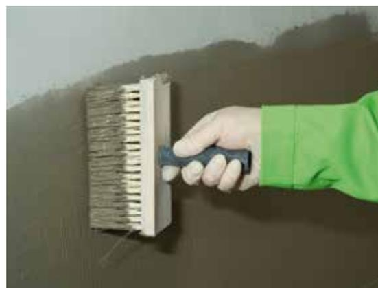
KÖSTER NB 1 Grey is applied using a coarse brush. Make sure to brush up and down as well as left and right in order to close all pinholes.
