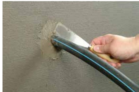
The pipe penetration is now waterproofed. In order to protect the waterproofing the area around the pipe or cable is plugged with KÖSTER KB-Fix 5.
