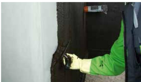
The first layer of KÖSTER Deuxan® 2C is applied, in this case by trowel. Surface profiles and unevenness up to a depth of max. 5 mm are filled with a scraped layer of KÖSTER Deuxan® 2C.
