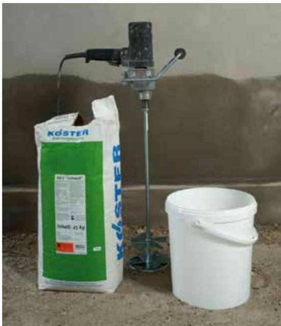
One bag (25 kg) of KÖSTER NB 1 Grey is mixed with 8 l of water. The water is placed in a mixing container of sufficient size.
