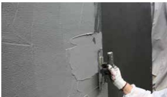
*KÖSTER NB 4000 waterproofing is safe and easy. Backfilling permitted after approx. 24 hours.*
