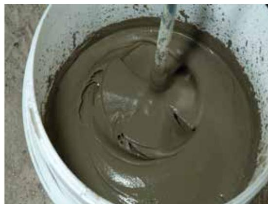
The powder is added in portions while continually mixing using a slowly rotating electrical mixer with a suitable mixing paddle. Mixing time is 3 minutes.
