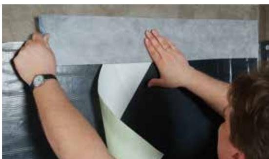
The upper edge of the waterproofing layer should end approx. 30 cm above grade and be covered with a cold self-adhesive KÖSTER Butyl Fix-Tape Fleece. This tape can be plastered over.
