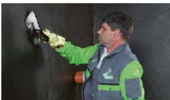
The second layer of Deuxan® 2C is applied shortly after the first layer of KÖSTER Deuxan® 2C.
