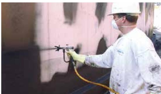
KÖSTER Deuxan® Professional is similar to KÖSTER Deuxan® 2C but specifically designed for spray application with a suitable spraying device. Spray application provides a very high productivity which makes it attractive for professional contractors and for larger objects. It requires knowledge of the pump and the spraying process. The spraying equipment has to be tested and fine tuned before commencing work.
