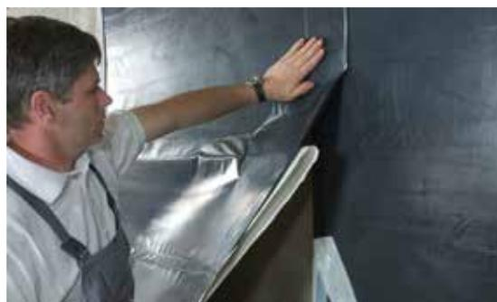
The area is waterproofed with the membrane. Membranes must overlap by approx. 10 cm.
