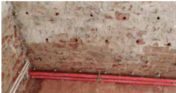
Exterior brick wall
