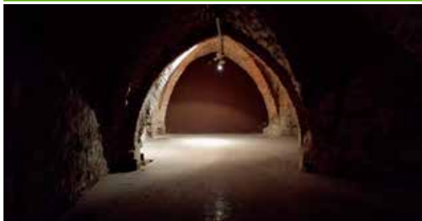
Historical vaulted cellars
