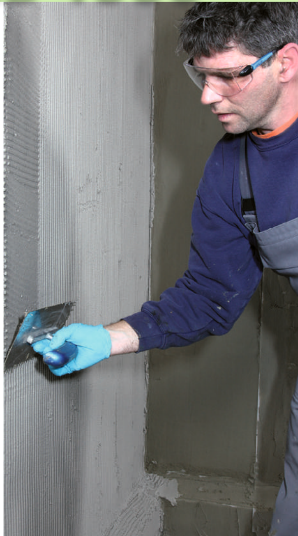
Internal waterproofing
