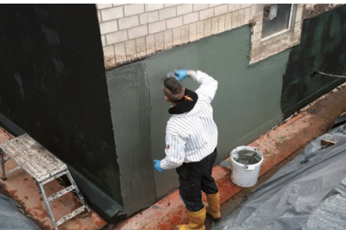
External waterproofing
